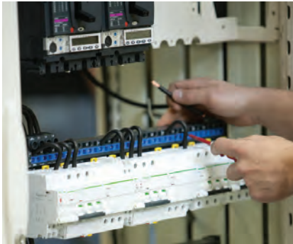
Fig. E30: Assembly of a final distribution switchboard with fixed functional units (Prisma Plus G)
